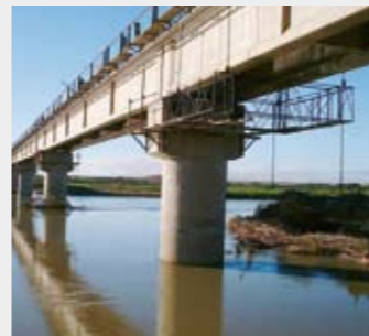
Ernest Oppenheimer Bridge (ZA)
