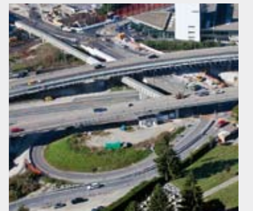
Highway Bridge A1, Bern (CH)
