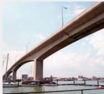
Itchen Bridge, Southampton (UK)
