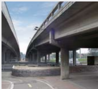
Two Bridges in Bogotá (CO)
