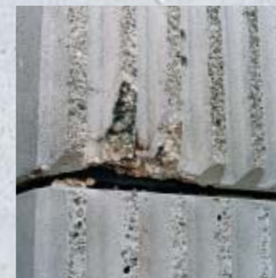
Cracking caused by incorrect handling or fixing of precast panels.
