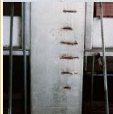
Reinforcement corrosion following reduction of the passivating concrete alkalinity by carbonation.
