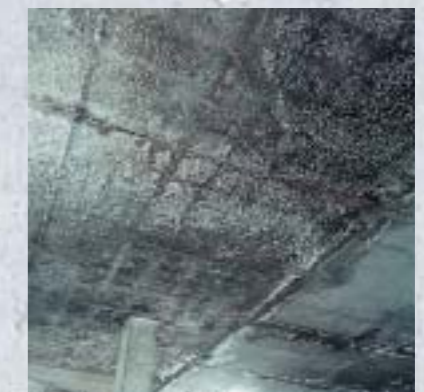
Freeze/thaw effect on a parking structure.
