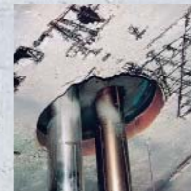
Chemical attack (and subsequent reinforcement corrosion) on a factory roof.
