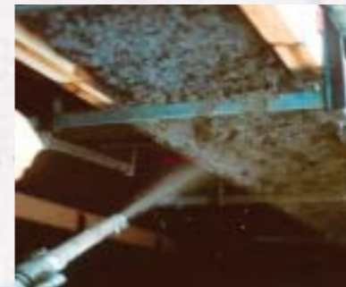
Spray application for test under live dynamic loading.
