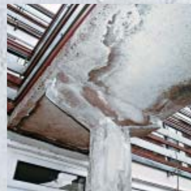
The damaging effects of steel corrosion accelerated by chloride ingress from deicing salts.
