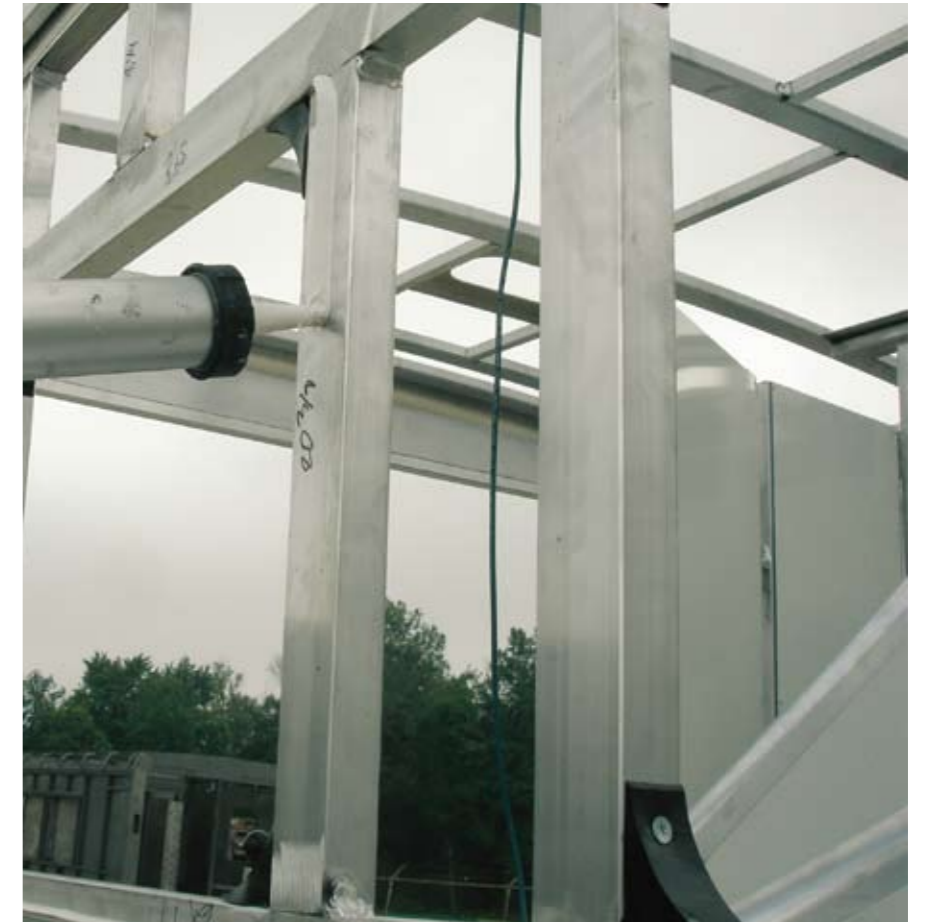
Bonding with Sikaflex®
