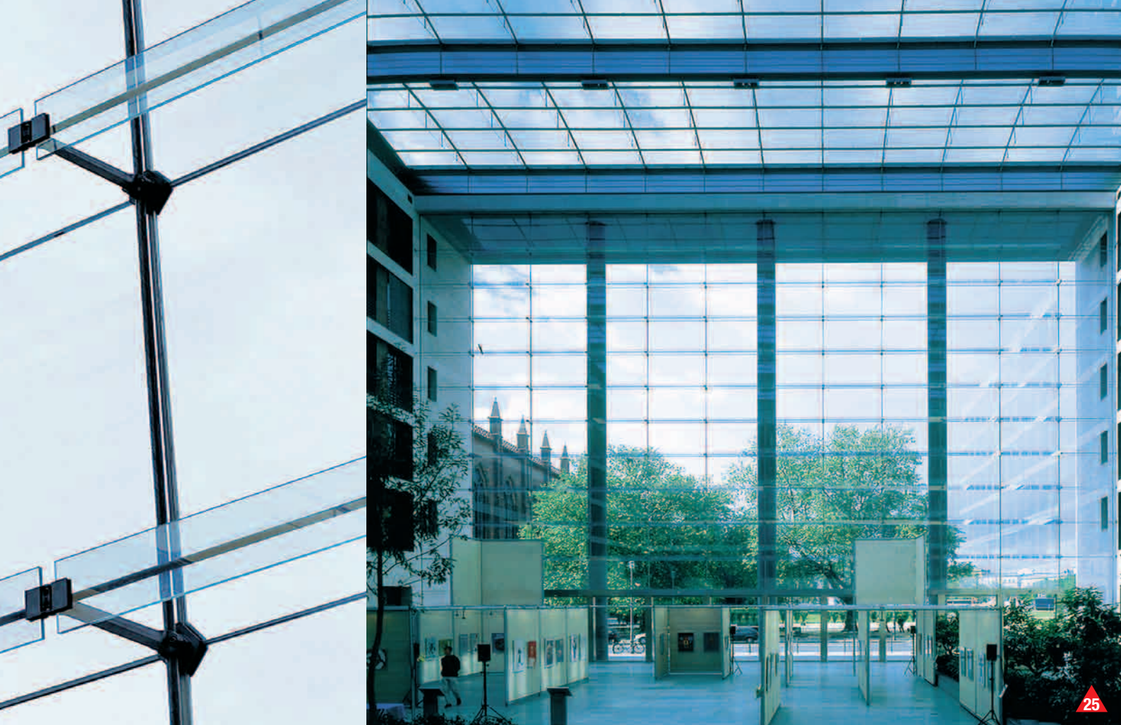
Extension of State Department, Berlin, Germany; design of glass facade: James Carpenter Design Associates
