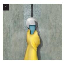
Substrate preparation by means of sandblasting, grinding etc., followed by vacuuming.
