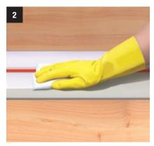
In case of dirt clean the surface of the **Sikadur-Combiflex**° **SG** tape with a dry or wet cloth. Use water and **no solvent** for cleaning.
