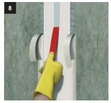
Remove the red middle strip and the masking strips on both sides to ensure a neat and precise detail.
