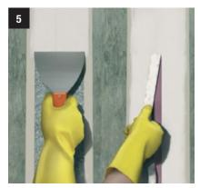
Apply the **Sikadur®-Combiflex® CF** adhesive on the left-hand and the right-hand side of the joint. Then remove masking strip.
