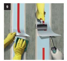
Connect tape ends by hot air welding.
