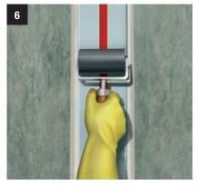
Press the **Sikadur-Combiflex** $^{\circ}$  **SG** tape without trapping air into the adhesive by using a suitable roller. The adhesive should be squeezed out on both sides by  $\sim$  5 mm.
