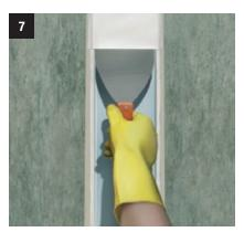
Apply the **Sikadur®-Combiflex® CF**Adhesive on the tape.
