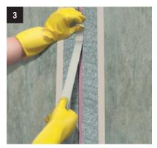
Use masking strips to cover the joint.
