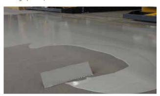
With such benefits, the obvious unique selling point is an ultra-fast system build up without preparing the substrate through shotblasting. The combination of SikaScreed® HardTop, Sikafloor®-140 W Troweling Primer and Sikafloor®-151/-161 in a timeframe of 48 hours provides at least the same bond strength as a conventional build up but without having an extra step of preparing the fresh installed mortar before coating.
