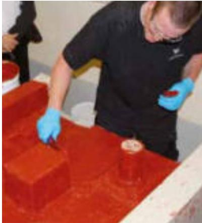
The unique – Sika MTC technology was developed using Sika's own custom pre-polymers and gives liquid polyurethane moisture triggered curing. It means no CO<sub>2</sub> outgassing in contact with water
