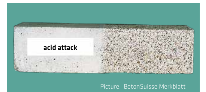
Acidic solvent attacks which dissolve calcium compounds out of the hardened cement matrix can be caused by acids, exchangeable salts, vegetable or animal fats or oils. Degradation of the concrete usually occurs very slowly.
