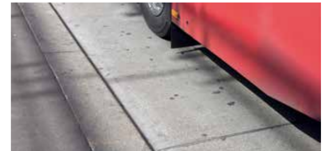
Concrete roadways and other publicly accessible areas, especially those experiencing high volumes of traffic or concentrated loads, are subject alongside high mechanical burdens also to strong abrasion, often presenting the risk of a smooth, slick surface.
