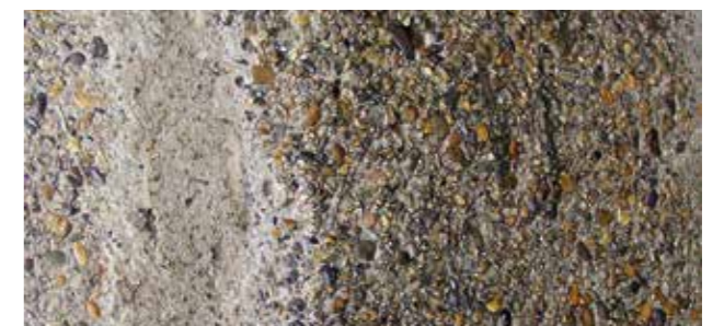
Due to continuous exposure, the cement film is eroded in an initial step, and thereafter larger and larger aggregates are rubbed, knocked or washed out of the hardened cement paste
