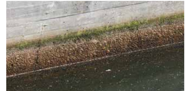
Heavy leaching and damage to the structural concrete are observed particularly in the water splash zone of biological treatment basins.
