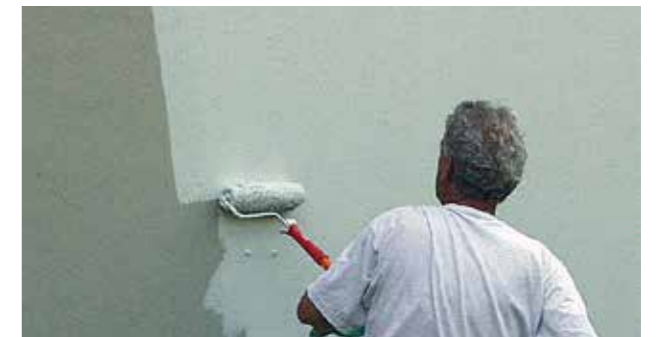
Epoxy resin-based protective coatings are applied over the entire surface following reprofiling of the concrete surface with sulfate-resistant repair mortar enhanced with synthetic material.
