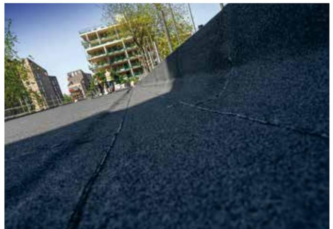
**Do not fill the joints with trowel, spatula or other tool,** because the reinforcement of the membrane can be affected, weakening it. In addition, the upper protective layer is removed and the reinforcement can be left exposed.
