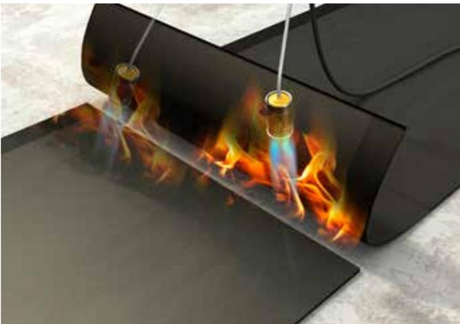
Whereas the lateral overlaps require adhesion zones free of grit, at the end overlaps the mineral-coated surface must be heated with a certain persistence so that melting consequently takes place over an area corresponding to the width of the overlap, with consequent melting of the bituminous mastic underneath.
