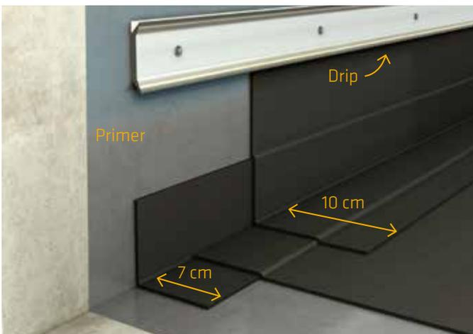
Along the perimeter of the roof and on the flat, the membrane should be bonded completely to the substrate. Same when applied with slopes higher than 15°: the membrane must be mechanically attached at the top.
