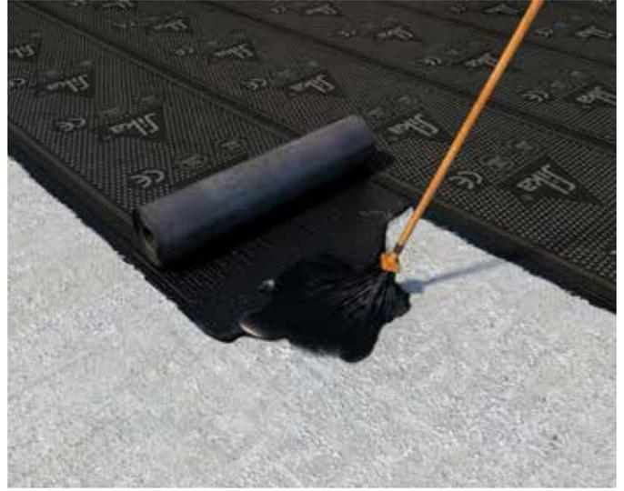
Apply the hot melt at the correct consumption to the prepared surface. The application must be done uniformly across the surface with a suitable spreader (a mop is widely used). The membrane must be laid immediately after while is still hot. Press the rolls from the center to the border to avoid the bubbles. The hot melt can also be used to seal the overlaps.
