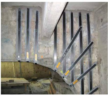
Sika CarboDur® strips and CarboShear L plates bonded to the concrete structure.
