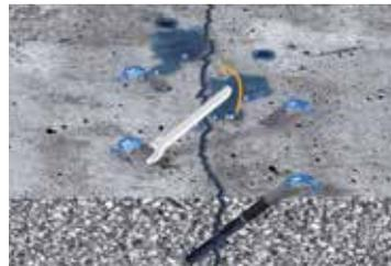
2. Install the mechanical packers.
