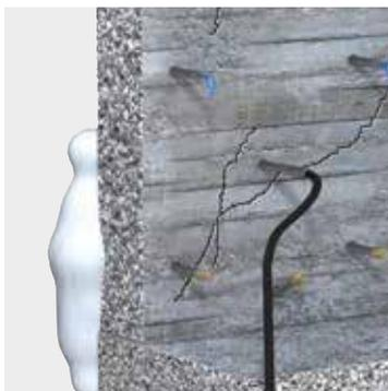
■ Grid injection (into the surface for larger areas e.g. Honeycombing or poor concrete compaction etc.)
