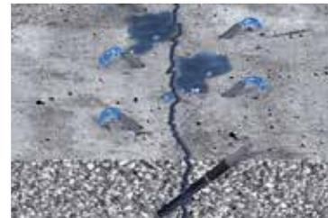
3. Fix the non-return valve on the first packer and start the injection process.
