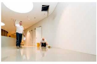
**STEP 4.** A wide selection of liquid resin products is available in an almost unlimited amount of colors to address many types of use. Decorative flakes or anti-slip aggregates may be broadcasted into the wet surface.
