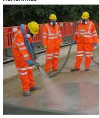
For durable crack-bridging protection of bridge decks.
