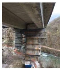
Protecting the embedded steel reinforcing bars against corrosion using hybrid technology (Induced Current Cathodic Protection & Galvanic Cathodic Protection).
