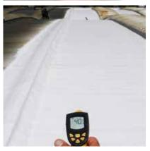
If applied in white (RAL 9016) color, the membrane systems provide excellent solar reflectance property to roofs, which result in so-called cool roofs that increase reflectance and reduce both the heat-island effect and the cooling energy consumption of buildings.
