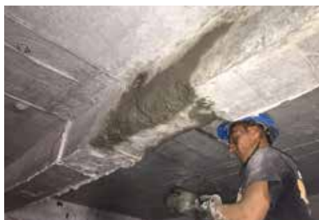
Concrete repair and refurbishment, Page 28
