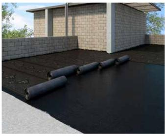
The overlaps must be sealed using other sealing product or by torch or welding.
