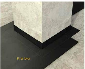
Apply again another piece of membrane on top of the first layer, now on the opposite side of the corner. In this case, the overlapping should have an angle of 45°.
