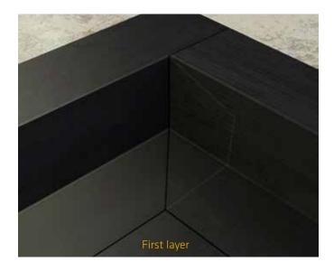
■ In case of a multilayer system, proceed with the application of the second layer following the same steps, but now starting on the opposite side of the corner.
