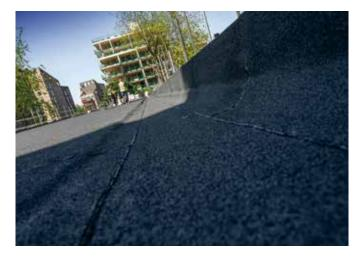
**Do not fill the joints with trowel**, spatula or other tool, because the reinforcement of the membrane can be affected, weakening it. In addition, the upper protective layer is removed and the reinforcement can be left exposed.
