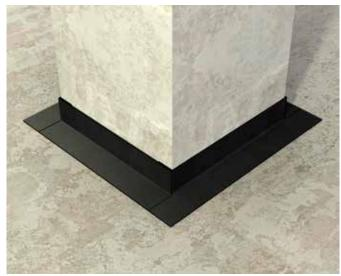
Cut another piece of the membrane enough to cover the entire corner angle. This must be done for all the corner joints. Then proceed with the application of the first layer of the bituminous membrane.
