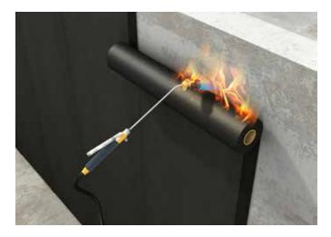
It may happen in the summer months that both, the membrane and the substrate, are so hot that they take a long time for sufficient cooling and full adhesion. In this case, the operator must carefully control the heating to prevent sliding of the membrane on the wall and fall.
