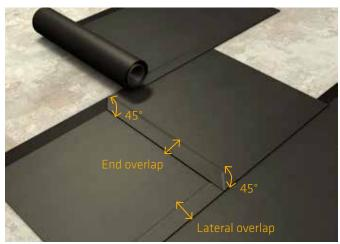
The overlaps must be welded with great care until a trickle of melted mixture about 1 cm wide can be seen coming out along the line of the overlap.
