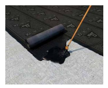
Apply the hot melt at the correct consumption to the prepared surface. The application must be done uniformly across the surface with a suitable spreader (a mop is widely used). The membrane must be laid immediately after while is still hot. Press the rolls from the center to the border to avoid the bubbles. The hot melt can also be used to seal the overlaps.
