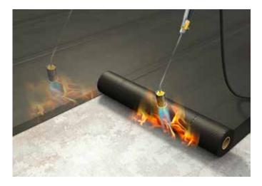
Flame heating must bring retraction of the film and flattening of the embossing, but heating the membrane any further can damage the polyester reinforcement, which melts at 260°C, causing retraction, undulations, curling or, in the most serious cases, puncture. Insufficient heating, on the other hand, can cause insufficient adhesion to the base between the layers or on the overlaps.
