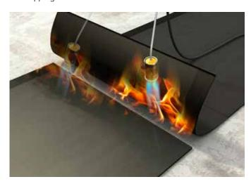
Whereas the lateral overlaps require adhesion zones free of grit, at the end overlaps the mineral-coated surface must be heated with a certain persistence so that melting consequently takes place over an area corresponding to the width of the overlap, with consequent melting of the bituminous mastic underneath.
