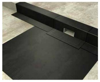
Proceed with the application of the first layer of the bituminous membrane, which cannot cover the drain area.
