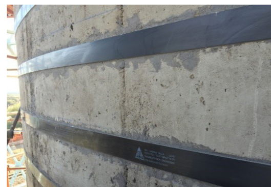
Contractor : Teichmann Structures
