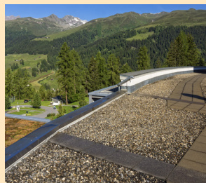
Gravel Ballasted Roofs
