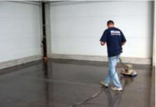
An impregnation is defined as the treatment of concrete to reduce the surface porosity and to strengthen the surface. The pores and capillaries are then partly or totally filled. This type of treatment usually also results in a discontinuous thin film of 10 to 100 microns thickness on the surface. This serves to block the pore system to aggressive agents.
