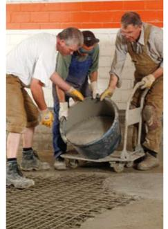
Typical recasting repairs, which are also frequently described as pourable or grouting repairs, are employed when whole sections or larger areas of concrete replacement are required. These include the replacement of all, or substantial sections of, concrete bridge parapets and balcony walls etc.
