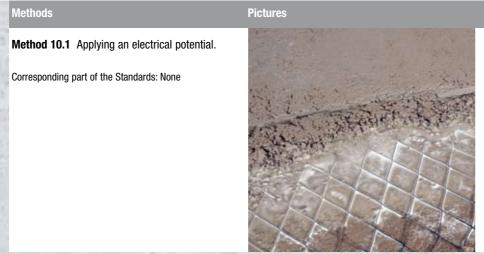
In Induced Current Cathodic Protection, the current is supplied by an external electrical source and is distributed in the electrolyte via auxiliary anodes (e.g. mesh placed on top of and connected to the reinforcing steel). These auxiliary anodes are generally embedded in a mortar in order to protect them from degradation. To work efficiently the system requires the surrounding mortar to have a resistivity low enough to allow sufficient current transfer.
