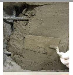
Traditionally the localised repair of concrete defects and damage has been undertaken using hand-placed repair mortars. Sika provides an extensive range of pre-batched, hand-applied repair mortars for general repair purposes and also for very specific repair requirements. These include lightweight mortars for overhead application and chemically resistant materials to protect against aggressive gases and
