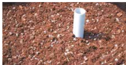
4. Laying of planting soil
