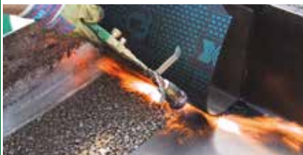
1. Application of DEFEND ANTIROOT in test device
