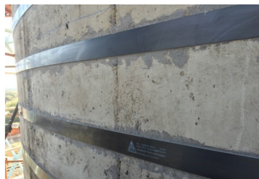
Contractor : Teichmann Structures
