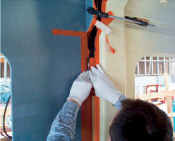
The joint between cab and main chassis, shown from the inside
