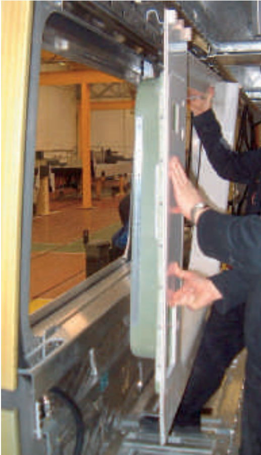
An interior panel is offered up prior to being fixed with Sikaflex®
