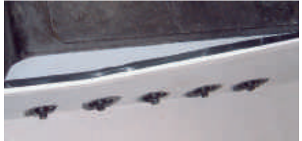
An interior joint is filled
