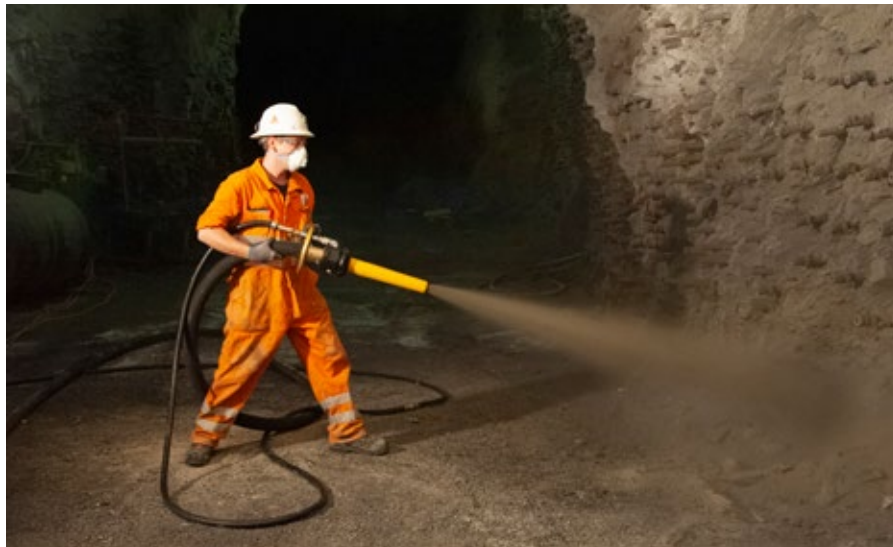
Fig 1.1: Shotcrete by thin flow process
