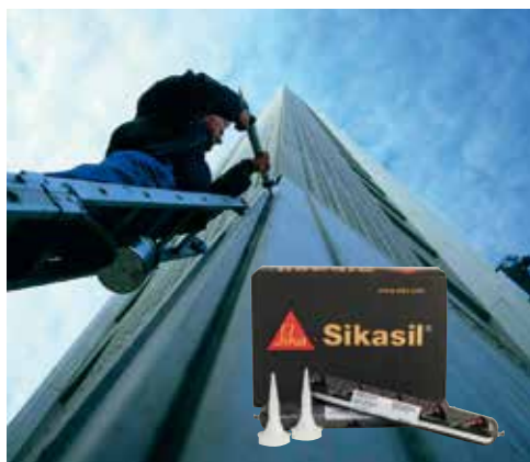
bottom: Gun application of 1-part sealants out of foil packs and cartridges (on-site application)
