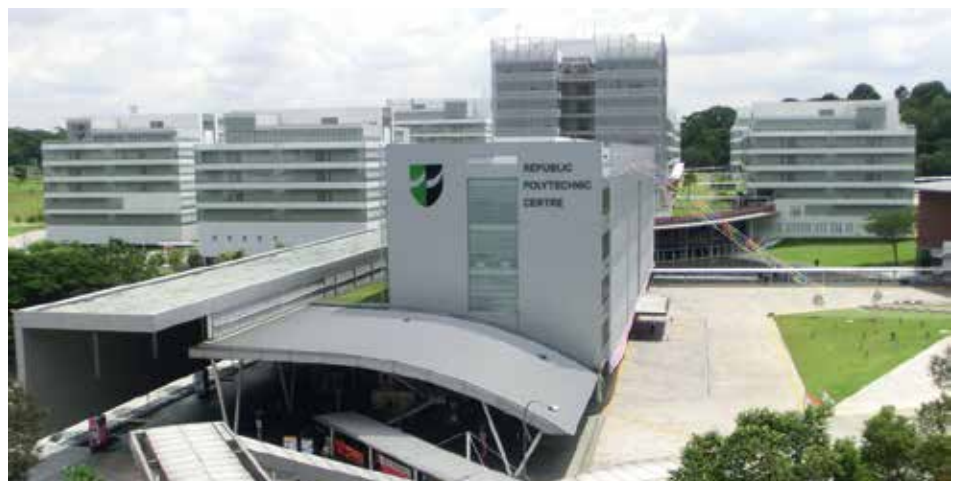
Republic Polytechnic Center, Singapore, 2006 Architects Fumihiko Maki, DP Architects; Sealed with Sikasil® WS-605 S, after >5 years no signs of streaking effect
