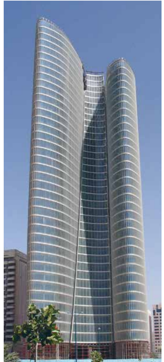
Adia Building, Abu Dhabi, 2006 Architects Kohn Pedersen Fox Associates PC Facade Schmidlin AG
