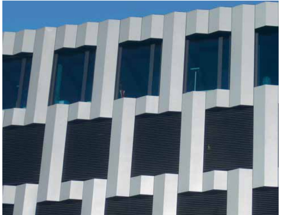
Office Building Zurich West, Zurich, 2013 Facade Yuanda Europe
