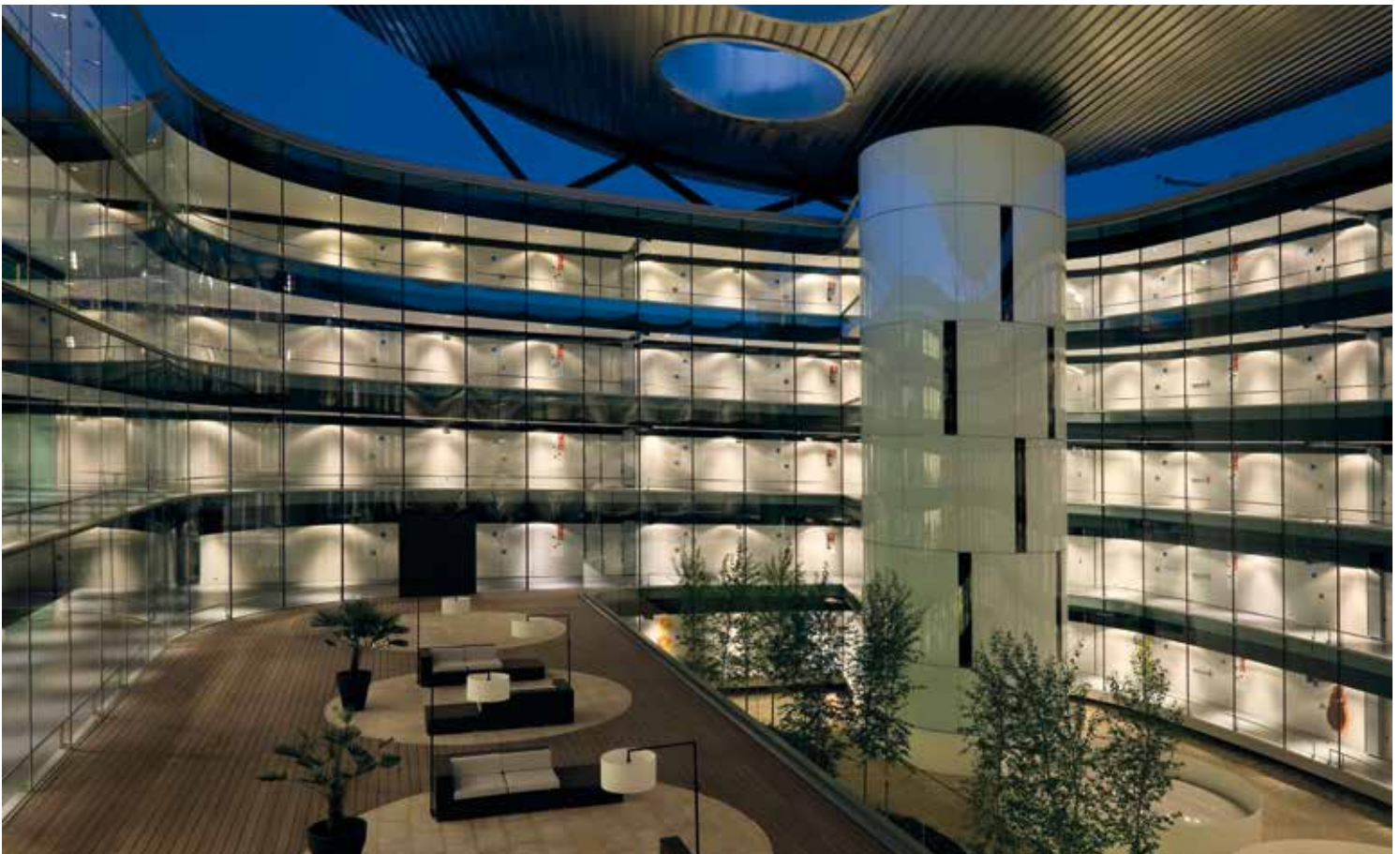
Hospital Rey Juan Carlos, Madrid, 2012 Architects Rafael De La-Hoz; Facade by Permasteelisa Spain; Curved Glass Cricursa
