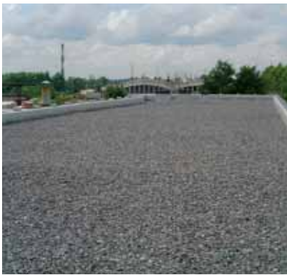
Gravel Ballasted Roofs
