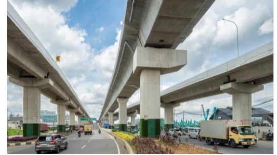
Road infrastructure project in Jakarta
