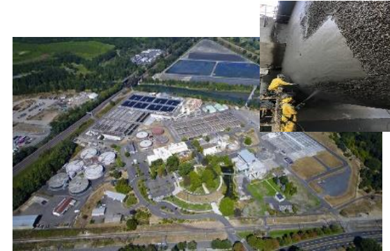
Waste water treatment plant refurbishment Oregon, USA
