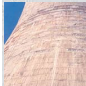
Quality control of the concrete. Core drilling on the wall.
