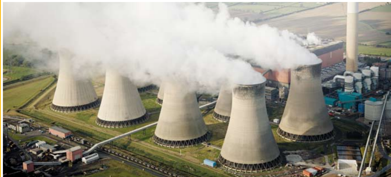
The severe combined exposure of multiple adjacent cooling towers and chimneys at power stations and industrial complexes.
