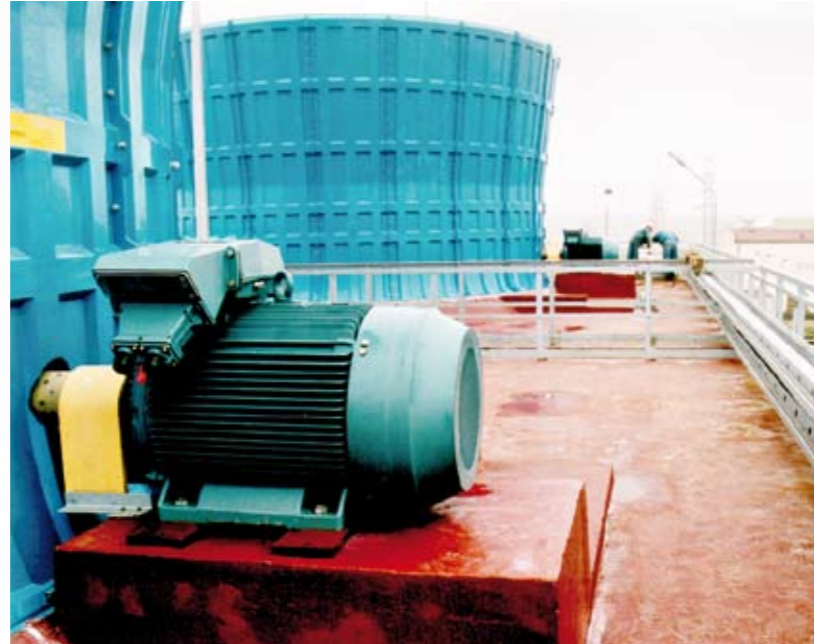
SikaCor steel coatings and Sikafloor concrete protection applied to ancillary equipment and surfaces.
