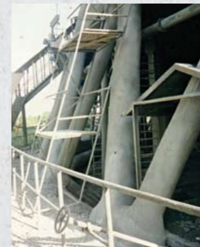
Difficult shaped support structures easily repaired and strengthened with SikaCem-Gunite 133.
