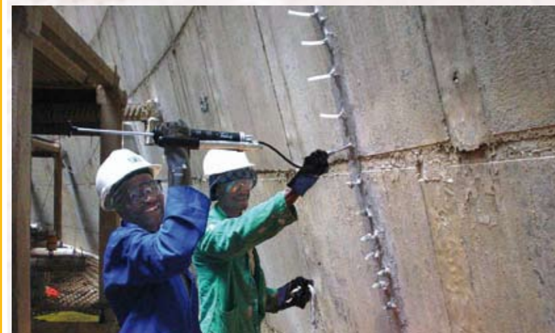
Structural bonding of cracks to restore structural integrity with Sika Injection resin.
