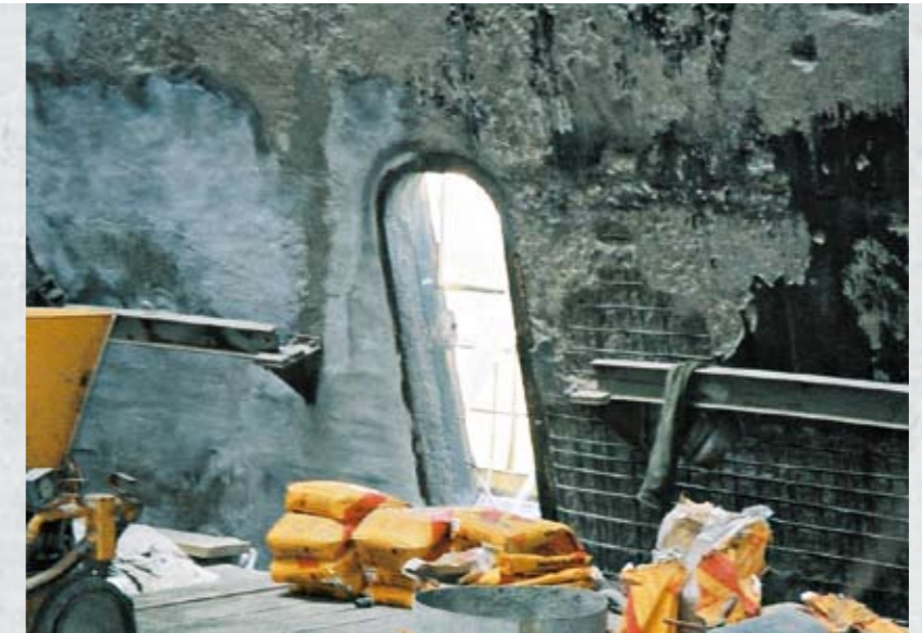
Sika Aliva dry spray equipment in operation applying SikaCem-Gunite 133 inside a cooling tower.
