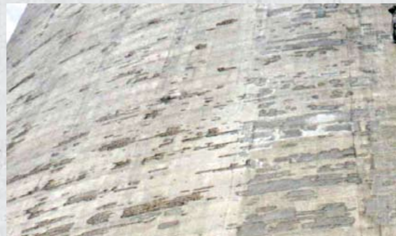
Hand applied local patch repairs completed on the external surface of a large cooling tower.
