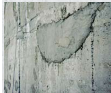
Hand applied Sika MonoTop repair mortar.
