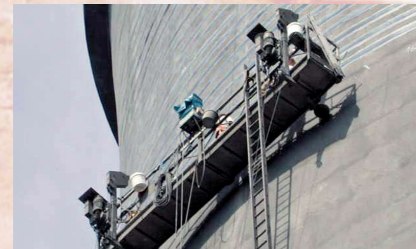
Sika CarboDur CFRP plates being bonded with Sikadur epoxy adhesive directly to the repaired external concrete surface at the top of a cooling tower for increased restraint.
