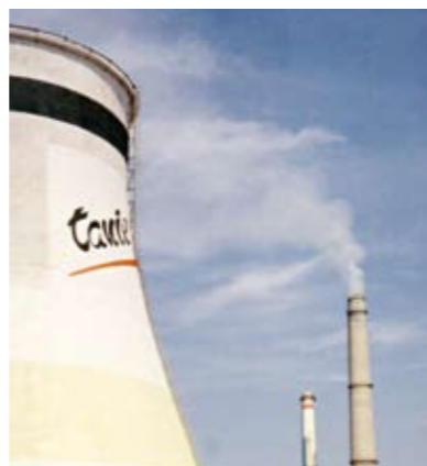
External coatings can be exposed to exhaust gases from adjacent chimneys.
