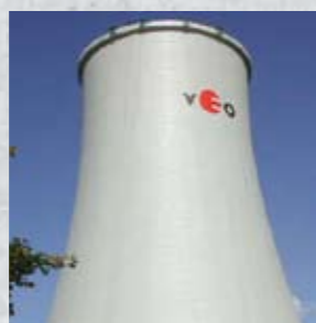
Autumn 2004, surface fully coated with Sikagard®-680 S concrete color.
