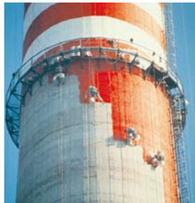
Abseiling specialists applying Sikagard-680 S.
