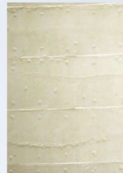
Icosit-2406 epoxy coating applied inside a cooling tower.
