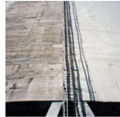
Locally repaired surface ready for levelling on the left and afterwards on the right.
