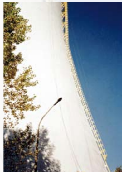
Galvanized steel ladders protected with direct application SikaCor coatings.
