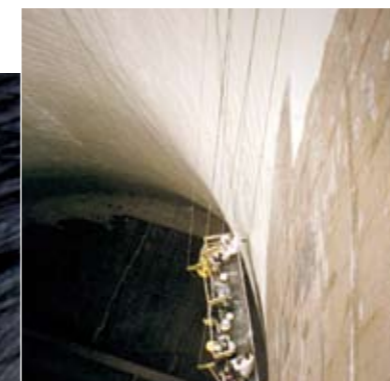
Severe internal exposure to aggressive gases and chemicals aggravated by direct UV light exposure and thermal variations at the top.
