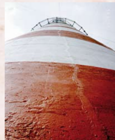
Crack-sealed with Sikaflex sealant and overcoated with Sikagard-680 S protective coating.
