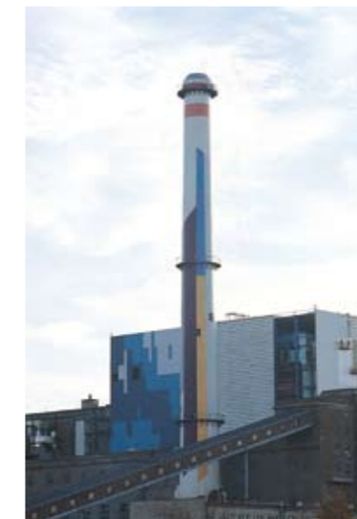
Creative possibilities in conjunction with using technically correct repair and protection are also possible with the advanced Sika systems.
