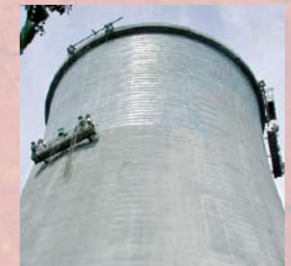
Easy application of the Sika CarboDur plates from powered access cradles.
