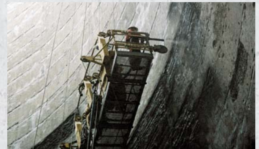
Internal application of Sika spray applied repair mortars in a cooling tower refurbishment.
