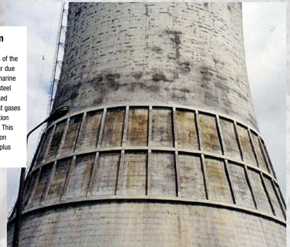
Carbonated concrete with spalling over corroded reinforcement accelerated by the steel being attacked by the acidic exhaust gases.
