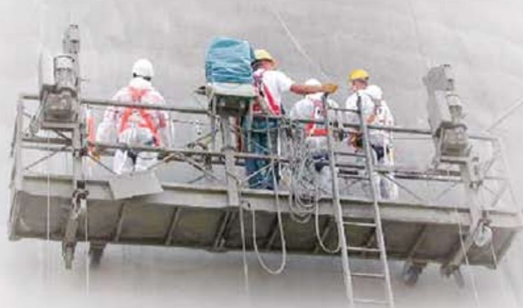
Specialist concrete repair and protection works in progress on the walls of a cooling tower.
