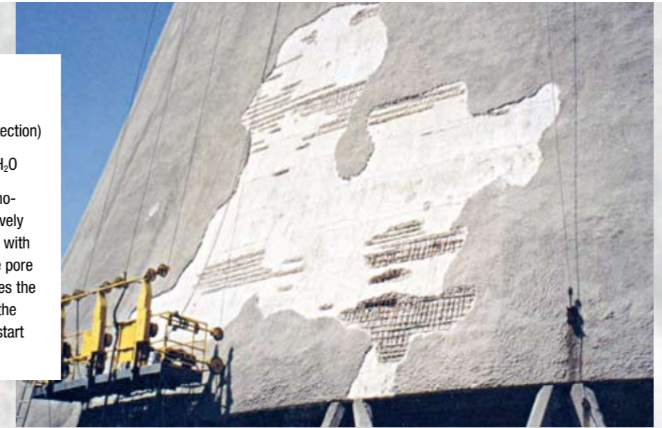
Concrete and previous overlay repairs spalling after carbonation has allowed the inadequately protected steel to corrode locally.
