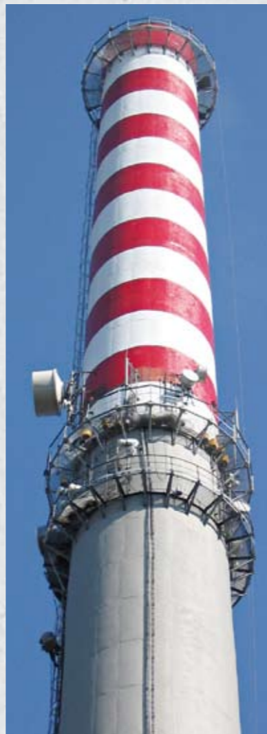
Aircraft warning colours to Zone 1 with high performance SikaCor EG 5 polyurethane top coat.
