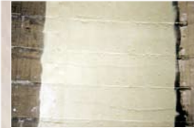
Close-up of the freshly applied Icosit 2406 epoxy protective coating system demonstrating excellent covering and sealing ability.
