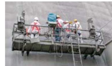
Application of Sika MonoTop-620 levelling mortar onto the patch-repaired concrete surface prior to coating.
