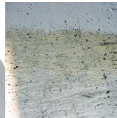
The concrete surface without pore filling and levelling.
