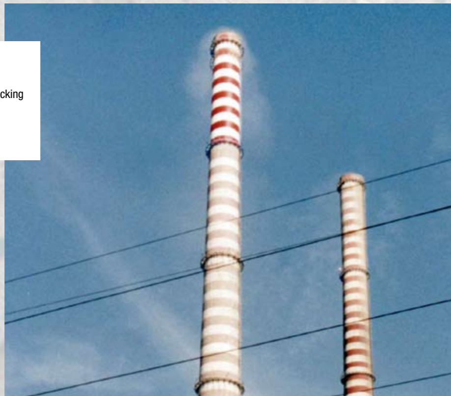
Chimneys in direct sunlight indicating variations in thermal exposure which are further exacerbated by the effects of the downward flow of hot exhaust gases during periods of temperature inversions.
