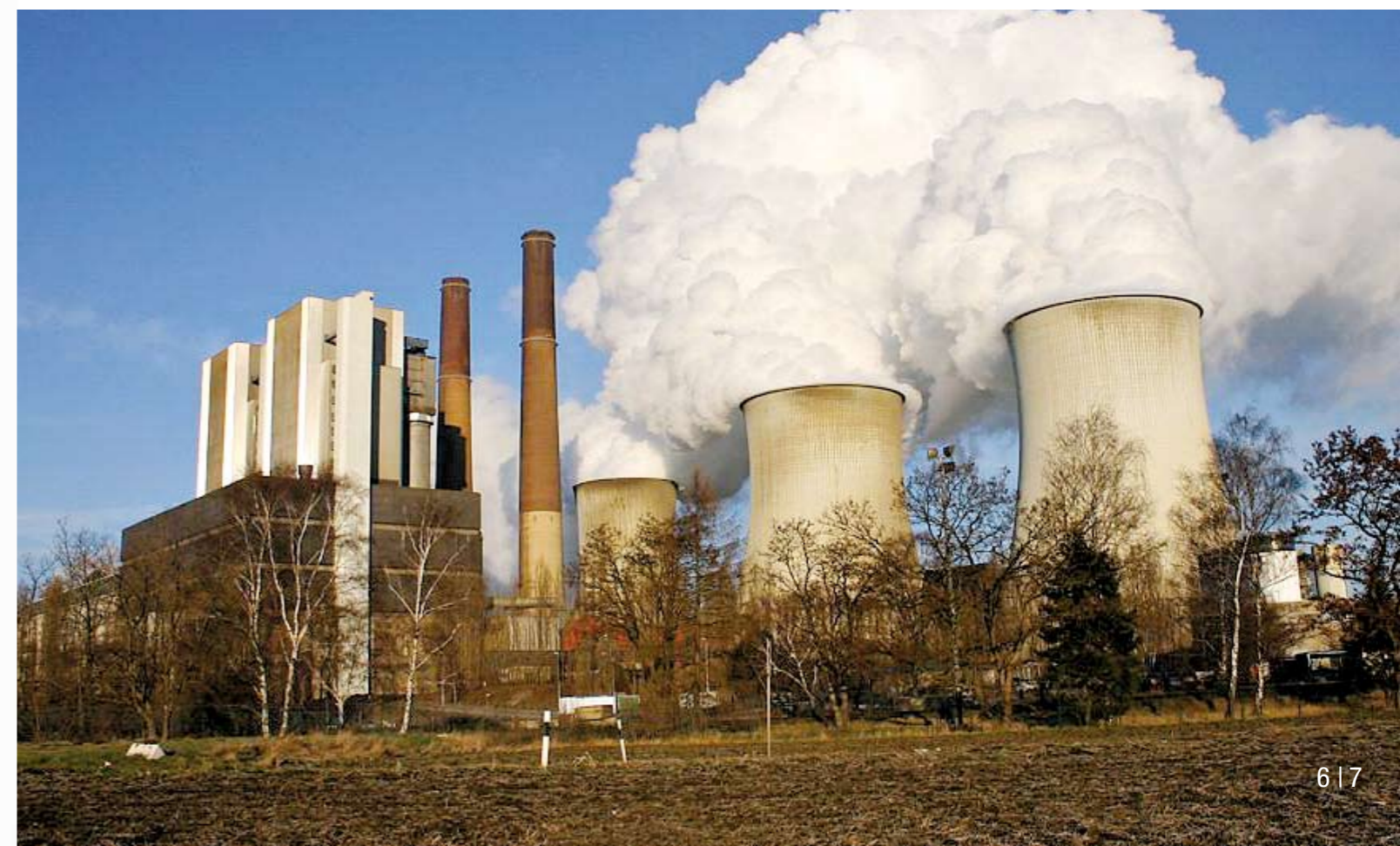
Chimneys and cooling towers in close proximity require technically correct repairs in accordance with EN 1504-9.
