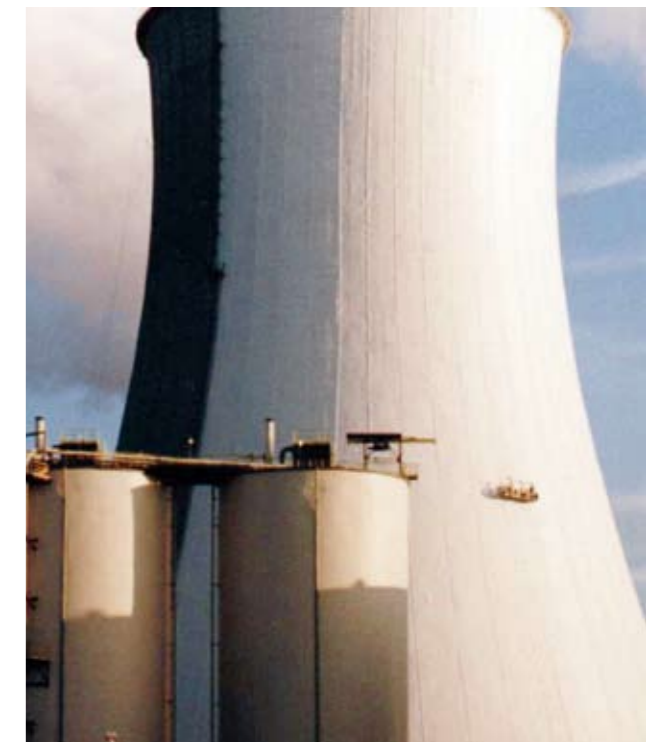
Sika protective coatings being applied to the external surfaces (all zones) of a cooling tower.
