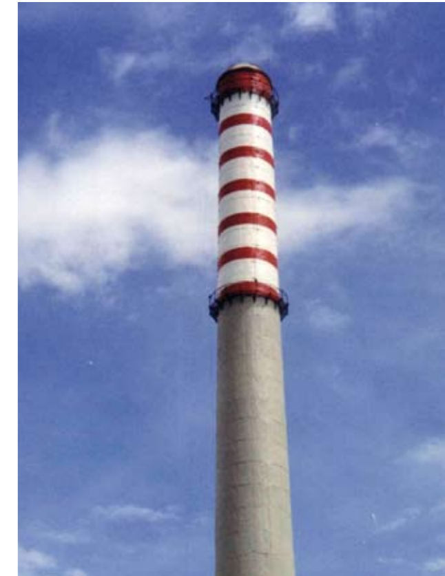
Aircraft warning colours using SikaCor EG 5 as the top coating in zone 1 of a concrete chimney refurbishment.
