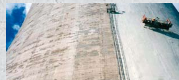
Protective coating being applied.
