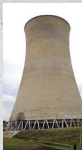
After 30 Years the concrete showed many cracks.
