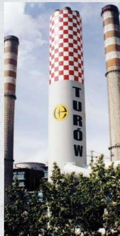
Adjacent chimney structures means that their surface exposure is increased in modern power plants and industrial areas.
