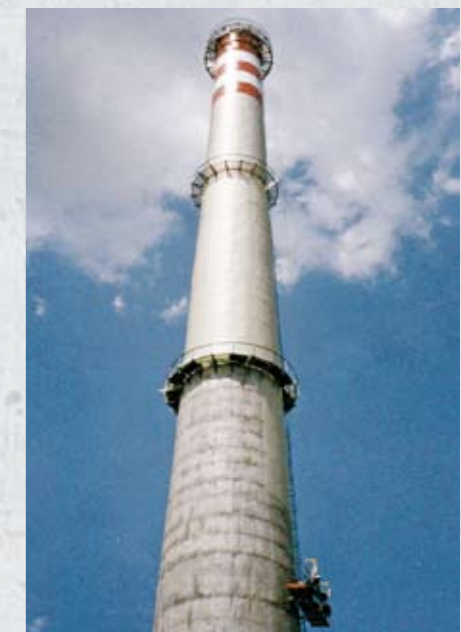
Typical chimney during the application of Sikagard protective coating systems, highlighting the different zones of external surface exposure and their protection requirements.
