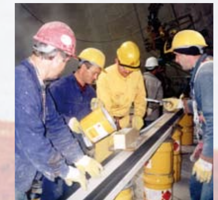
Sikadur adhesive application to the Sika CarboDur plate.
