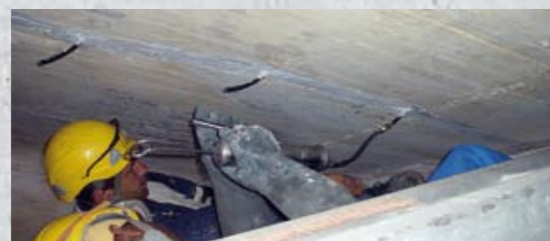
Crack Injection.
