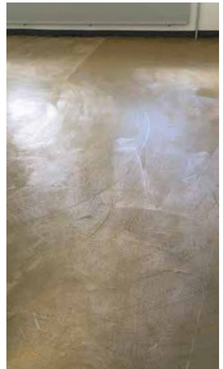
Floor substrate covered with adhesive.
