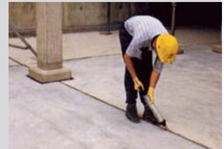
11 Sealing of Joints
