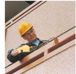
One-coat application of Icosit HS 6630 directly onto galvanised parapet railings
