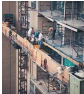
Application of Sika FerroGard-903 onto the prepared and repaired deck
