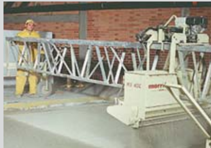
6 Mechanical Application of Dry Shake
