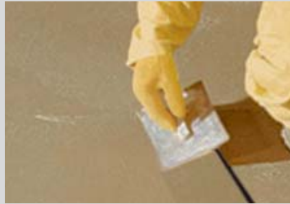
4 "Trowel Test" Is the concrete ready for the dry shake?
