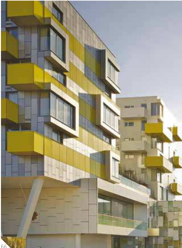
66 66 Lifelong Learning Centre, Barking, UK Architect: Allford Hall, Monaghan Morris (UK) Facade by Cladding UK
