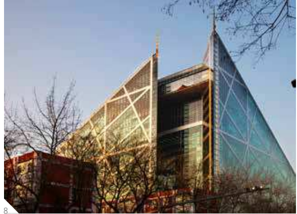
8 Park View Green Plaza, Beijing (2010) Consultant: ARUP Hong Kong Facade by Beijing Jianli (CN)
