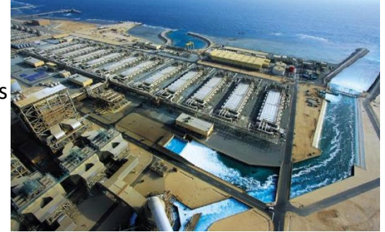
Vertical market approach Seawater desalination plant, UAE
