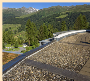
Gravel Ballasted Roofs
