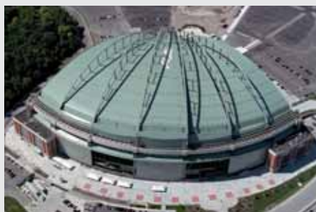
Miller Park, Milwaukee, USA
