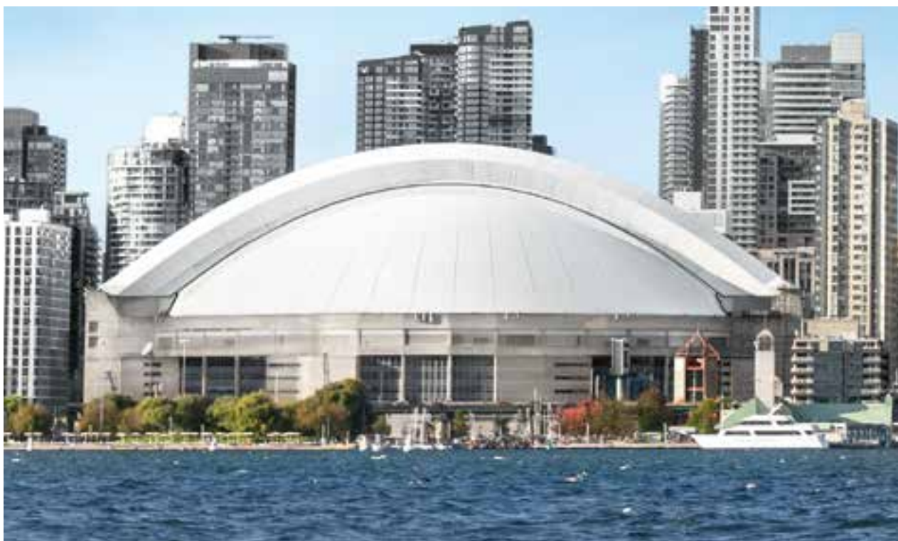
The Rogers Centre in Toronto, which was completed in 1989, was the first building in the world to have a retractable roof. No less than 41,000 m 2 of Sika Sarnafil membranes were used in its construction. All of this material was recycled when the building was renovated 30 years later, and the roof was once again sealed with a Sika Sarnafil system.
