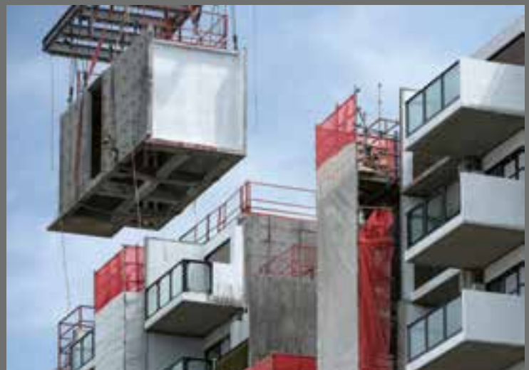
Avenue South Residence is the name of the world's tallest building to see the light of day thanks to modular construction. This high-rise is likewise being built in Singapore. By 2022, the twin towers will reach a height of 192 m and offer scope for more than 1,000 exclusive apartments. Special cranes are in place to lift the up to 30-ton modules into position correctly.
