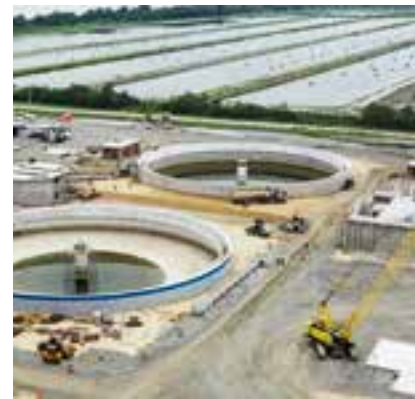
In Guayaquil, Ecuador, Sika is currently supplying products for a new wastewater treatment plant. One million apartments will be connected to the corresponding sewage system.
