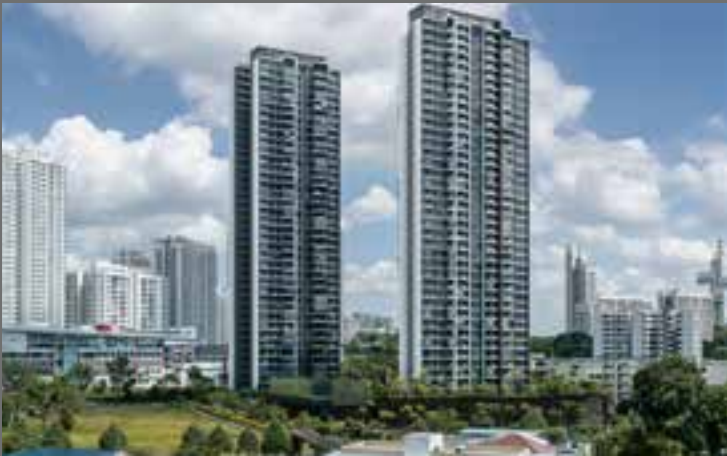
The twin towers of Clement Canopy in Singapore soar 140 m into the sky. 1,900 modules joined together make up the 500 apartments which form the supporting structure.
