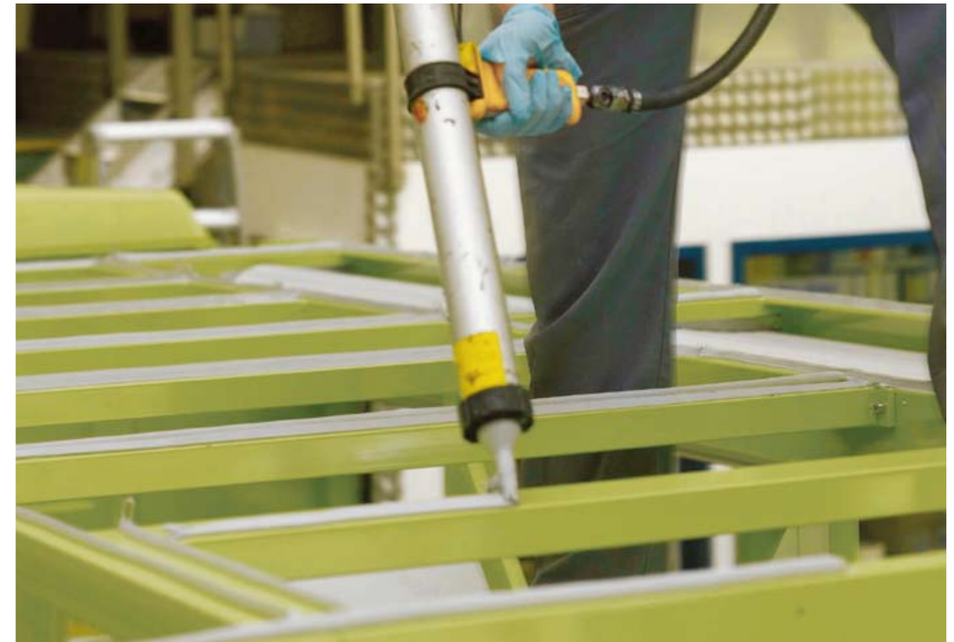
Application of the adhesive for roof panel bonding
