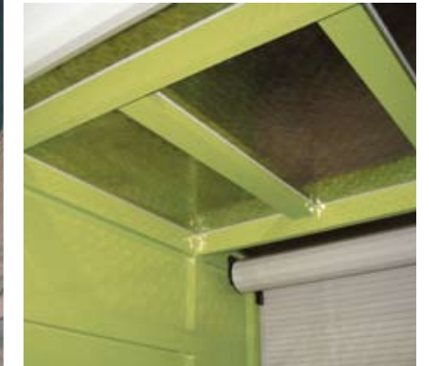
Sealed roof panel
